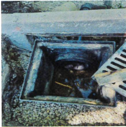
Storm box set and piped
