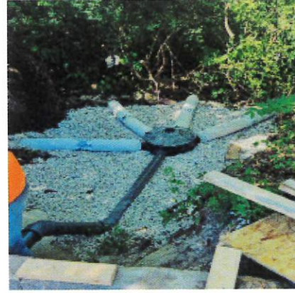
Detetion basin and ez drain outlets
