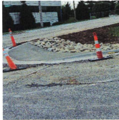
New Drainage Flume with Rip Rap
